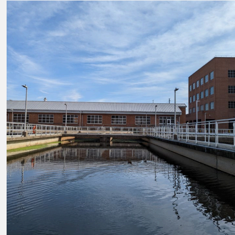
Wastewater treatment and combined sewer outfalls
