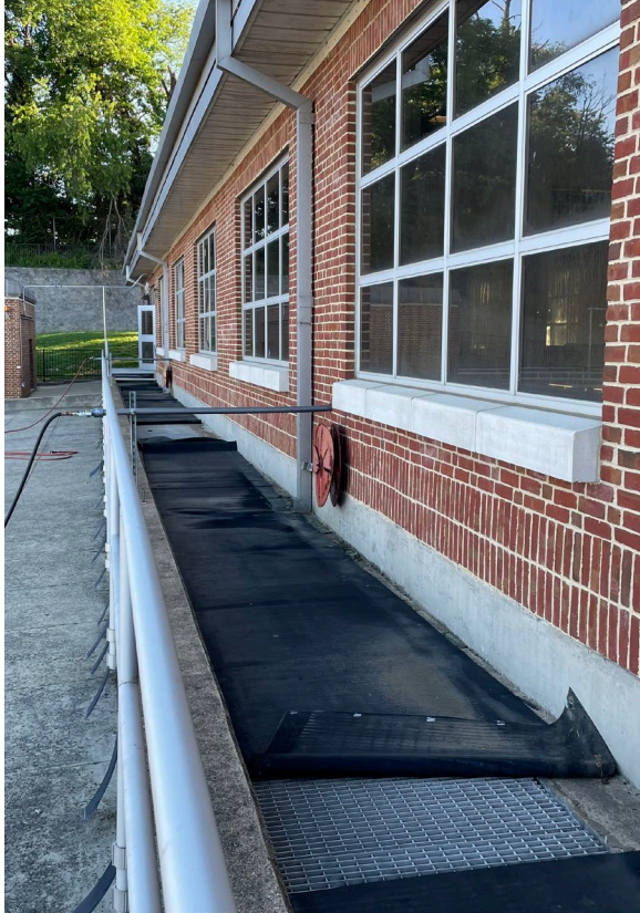
Repair concrete and install new covers over the primary effluent channel
