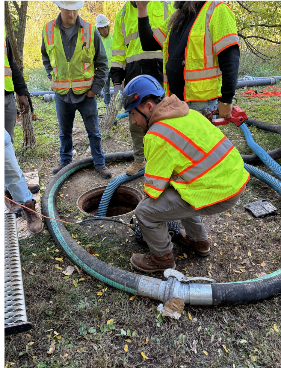
Potomac Interceptor Sewer Cleaning – Fall 2025
