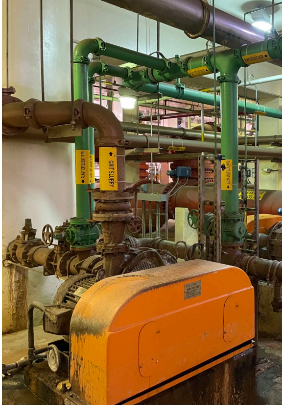
Replace two (2) vortex grit separators
