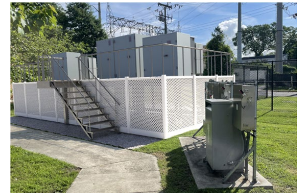
Install new electrical equipment to support new process equipment
