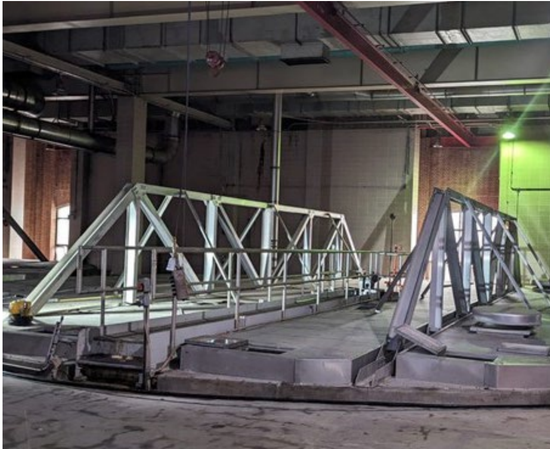
Existing Facility Upgrades
