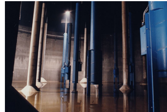
Decommission and demolish the existing gas mixing system and replace with hydraulic jet mixing
