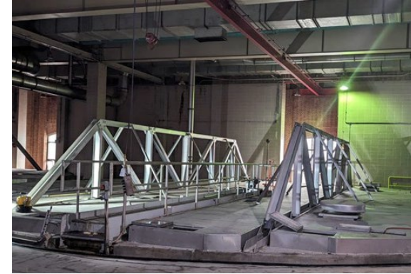
Fully refurbish gravity thickeners (3) (i.e., new rake drives, piping, scum collection systems, covers, & controls)
