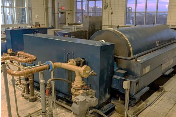
Replace dewatering centrifuges (3) & add a fourth unit
