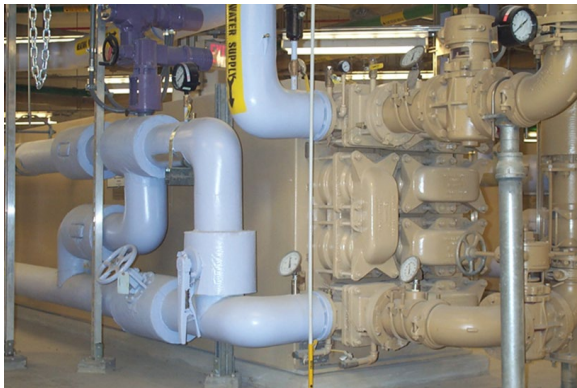
Replace digester heat exchangers (4) with larger units to provide all digester heating
