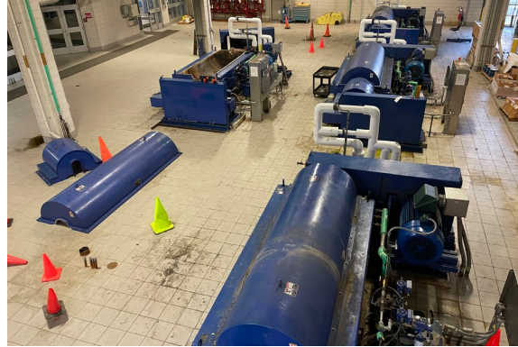
Replace thickening centrifuges and drive motors (4) and add a fifth unit
